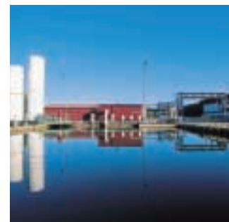
Toray is extending Torayca* production facilities at SOFICAR in France to satisfy long-term demand growth for carbon fiber. Equipment with a capacity of 1,800 tons/yr will begin operation in August 2004.
