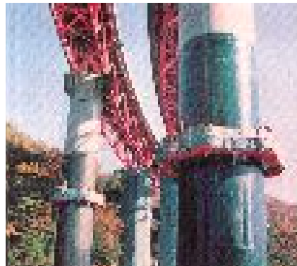
Bridge pier reinforcement
