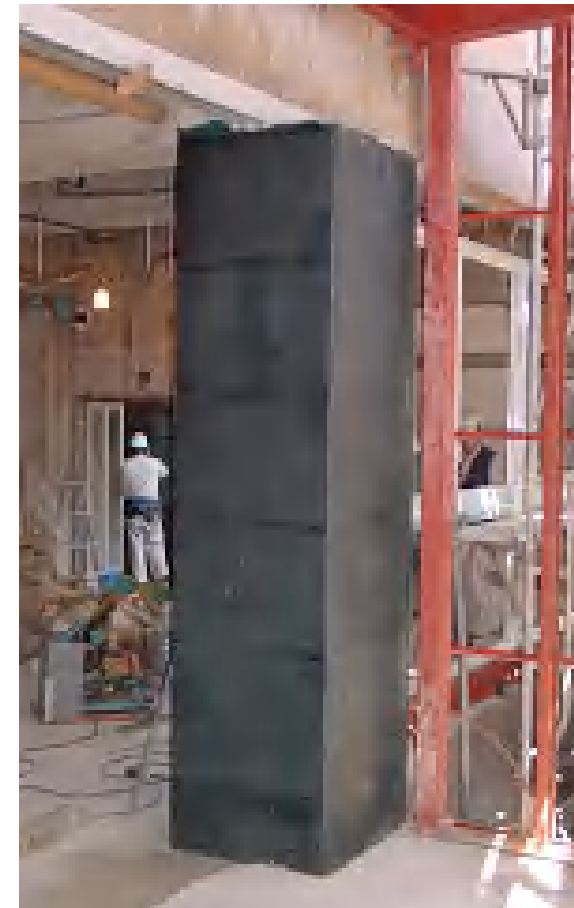
Pillar reinforcement
