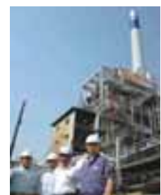
Power generation boilers at Toray Mishima Plant
