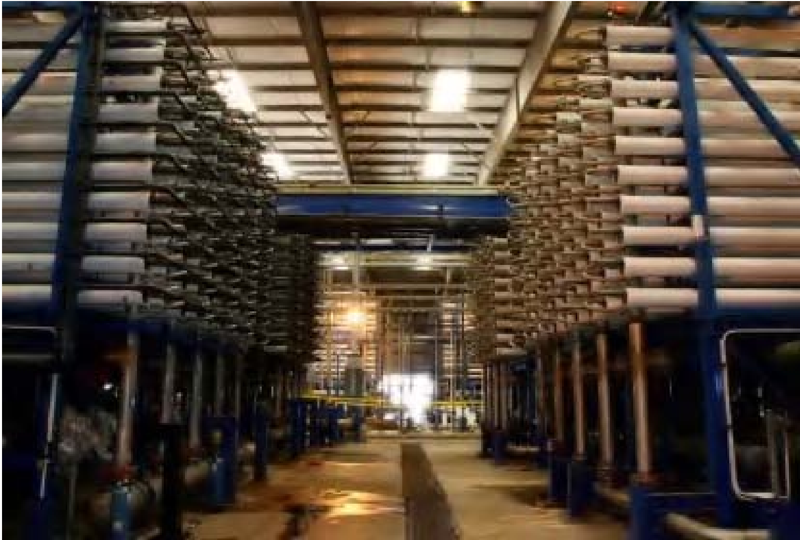
Trinidad & Tobago, the Caribbean Sea, Seawater Desalination Plant (Capacity: 136,000m 3 /d, Online: 2002)
