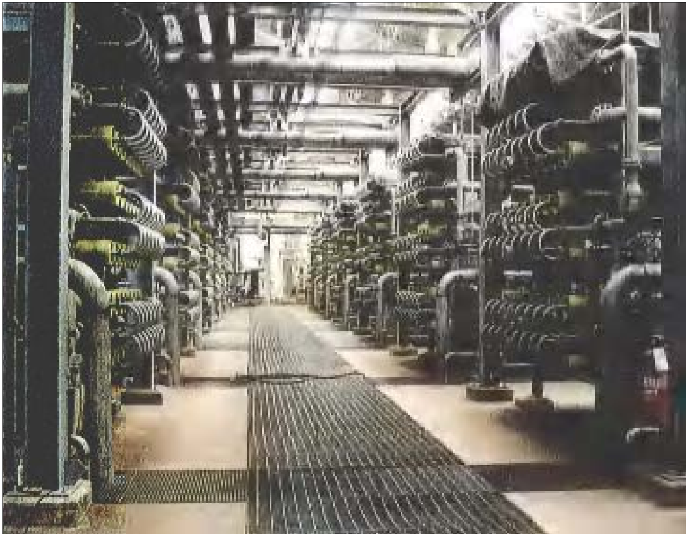
Brackish Water Desalination Plant for Petrochemical Industry
