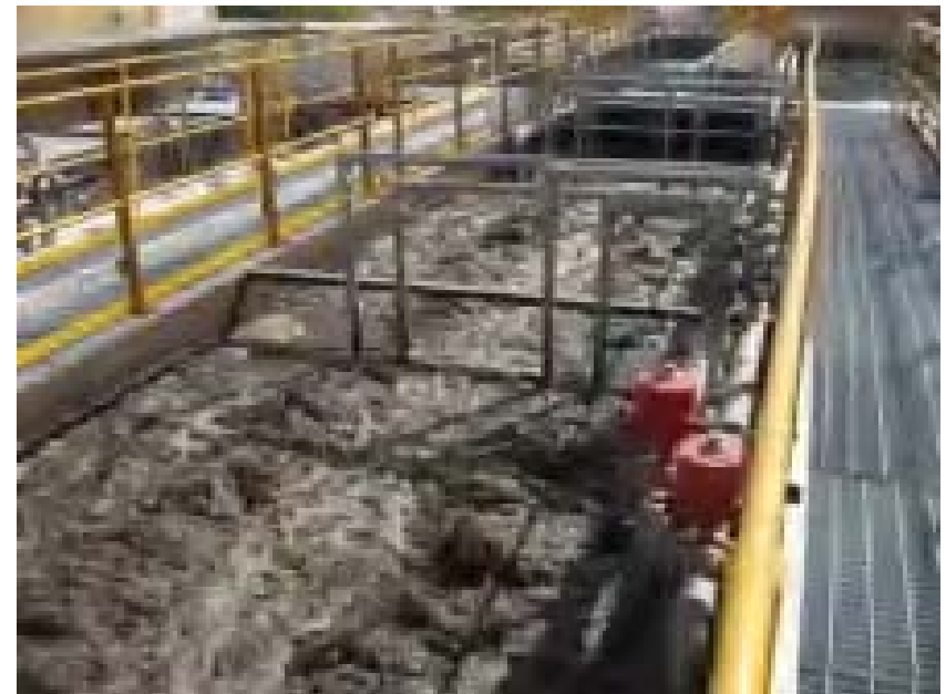
MBR Plant Overview
