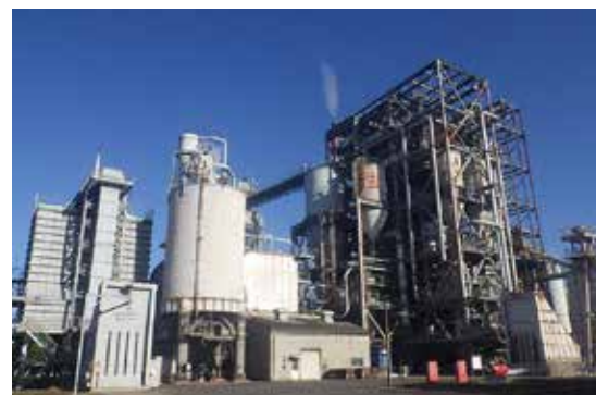
Facility for co-combustion of sludge fuel at Tokai Plant (Toray Industries, Inc.)
