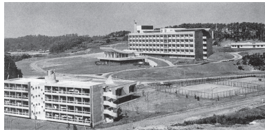
Completed Basic Research Laboratories (1962)
