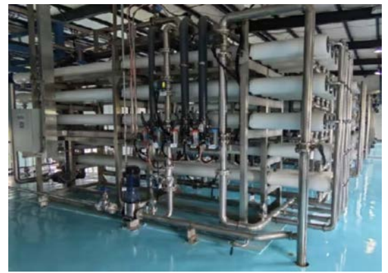
Dyeing effluent is reused at Toray Sakai Weaving & Dyeing (Nantong) Co., Ltd. utilizing Toray reverse osmosis membranes.
