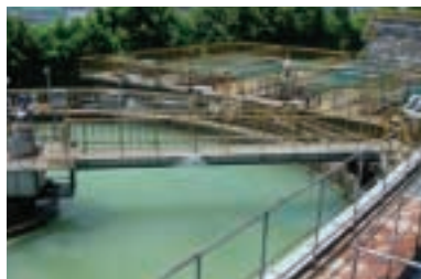
Wastewater treatment system at Okazaki Plant
