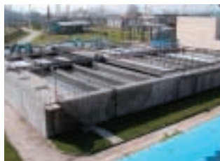
Toray Sakai Weaving & Dyeing (Nantong) Co., Ltd. Wastewater treatment system (China)
