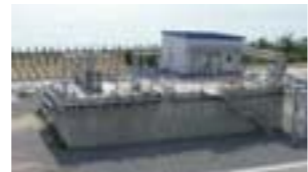
The Ehime Plant's new MBR treatment facility
