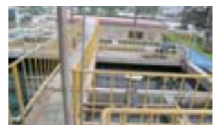
New wastewater treatment facility at TPSZ in China
