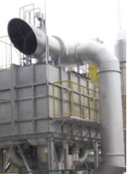
Regenerative combustion facility for organic exhaust gases installed at Toray Advanced Film
