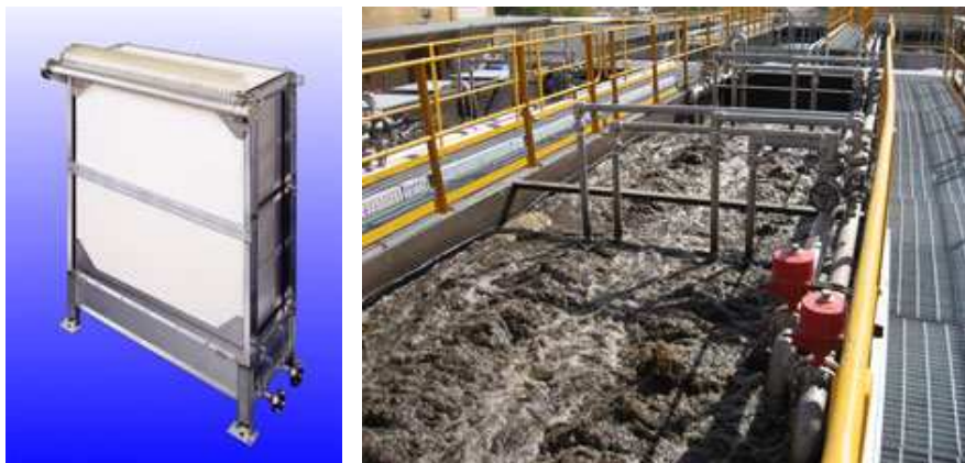
MF membrane modules for MBR (left) and the MBR plant in UAE (right)
