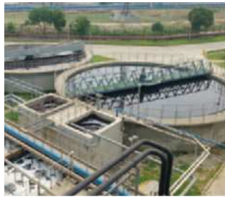
Wastewater facility at Toray Sakai Weaving & Dyeing (Nantong) Co., Ltd.
