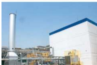
Cogeneration facilities at Toray's Okazaki Plant
