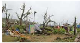
One of the first areas hit by Typhoon Haiyan, that suffered catastrophic damages to the water supply and sewers
