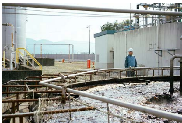
Wastewater treatment using the activated sludge method
