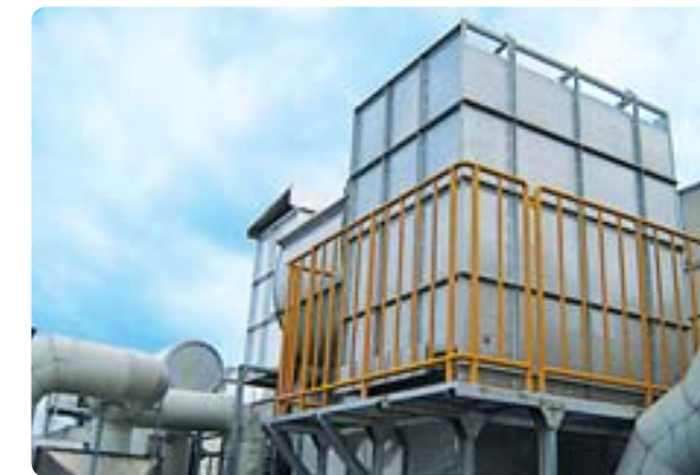
Organic exhaust gas direct combustion system at Toray Advanced Film
