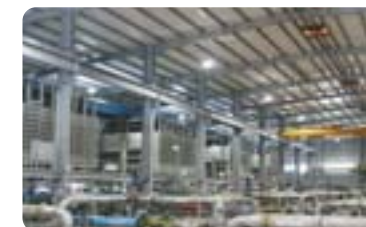
Seawater desalination plant in Singapore, using reverse osmosis membrane
