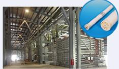
Singapore's largest wastewater recycling plant in the Changi region ©Sembcorp NEWater Plant, Singapore Upper right image shows Toray's ROMEMBRA® RO membrane elements
