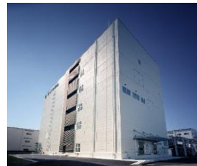
High-capacity plant for high-potency pharmaceuticals
