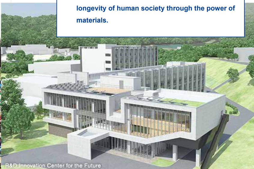
R&D Innovation Center for the Future
