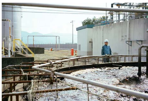
Wastewater treatment using the activated sludge method
